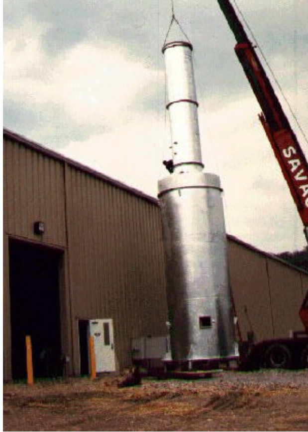
15,000 SCFM @ 2200F Thermal Oxidizer
