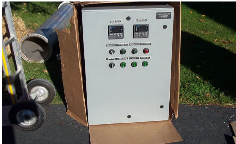
Typical HTT Control Panel
